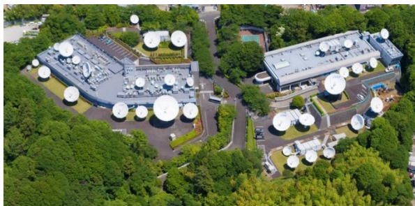
Primary Satellite Control Center – Yokohama Satellite Control Center (YSCC) : Numerous parabolic antennas pointing to satellites from 85E to 169E longitude. Large antennas over 4m in diameter totals to 29 * 3
