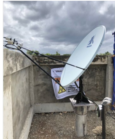
Protective walls against strong wind
