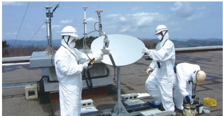
Installing satellite communication antennas in the disaster-affected areas
