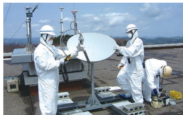
Installing satellite communication antennas in the disaster-affected areas
