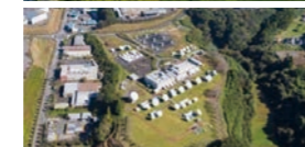
Back-up Station – Space Port East: Located in Hitachi-Omiya City of Ibaraki Prefecture, it has a total of 64 antennas*3
